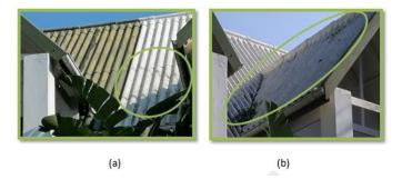
Figure 3: (a)-lichen growth on upper coated roof surface; (b)-lichen growth on lower coated roof surface
